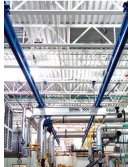
H.R. GREEN, WHICH JUMPED 160 SPOTS IN ENR'S LIST OF TOP DESIGN FIRMS, DESIGNED THIS LANDFILL GAS-TO-ENERGY FACILITY IN LAKE MILLS, IOWA.
